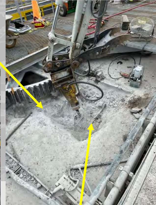
Embedded piece of Reaction Roller Base
