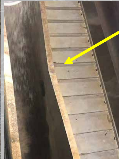
Impact damage to Gate #2
