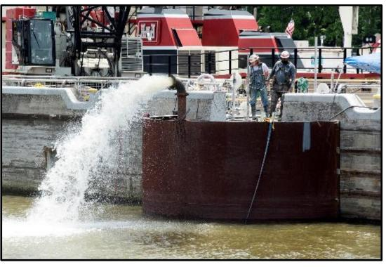
21 May 2021 – Maintenance workers pumping out water from a dewatering box to perform work in the dry.
