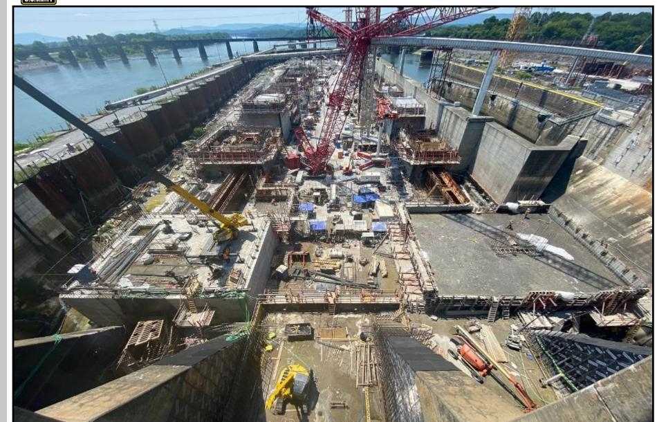
Looking downstream overlooking completed drilled shafts, monolith placed concrete, formwork, and rebar installation.
